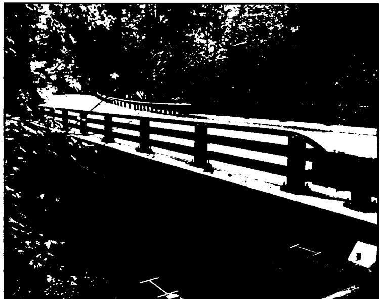
Cougar Creek Bridge No. 1409 completed in 2012.
