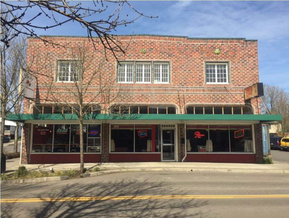
Photo 1: South primary façade
