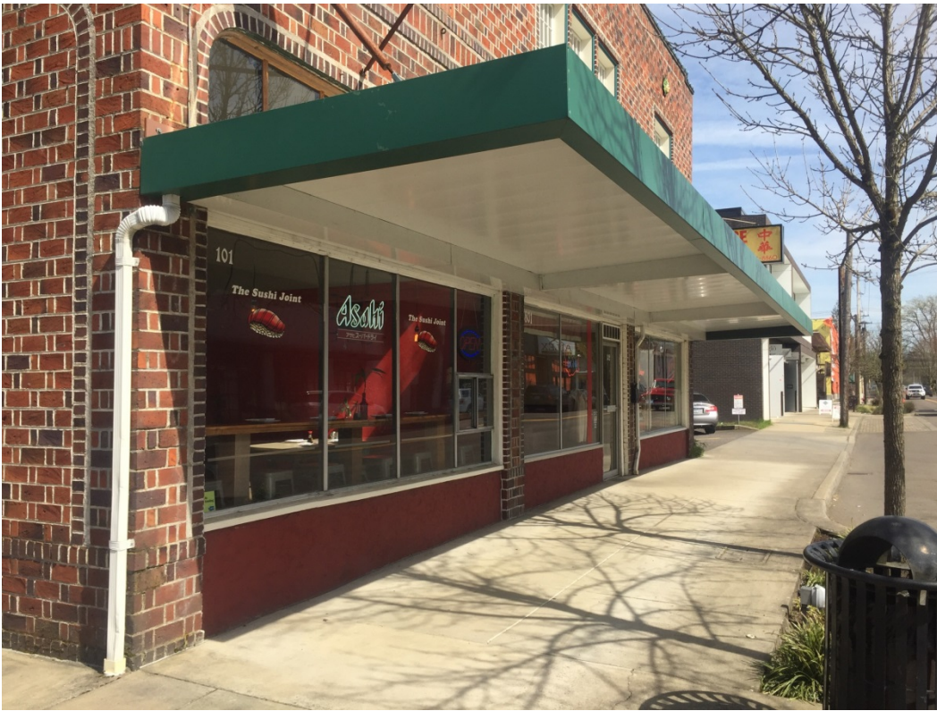
Photo 6: Detail of south façade, west end, showing window adapted for serving ice cream to customers on sidewalk
