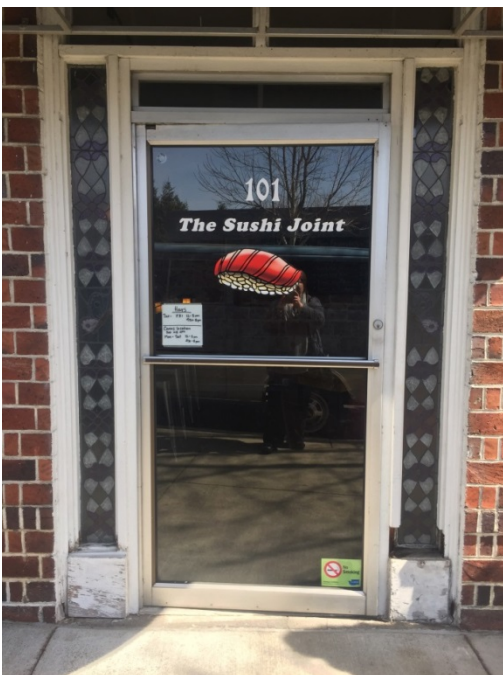
Photo 10: Detail of west façade showing entry to Sushi Joint
