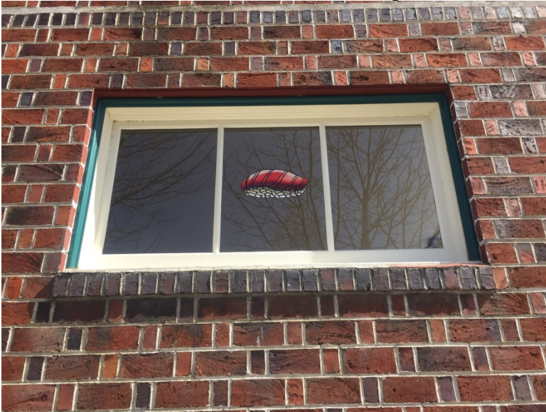
Photo 11: Detail of west façade showing window
