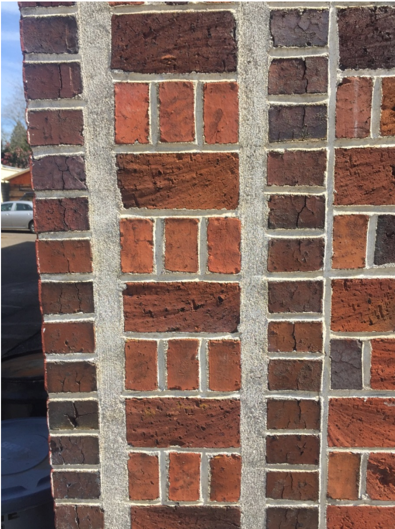
Photo 12: Detail of west façade corner brickwork
