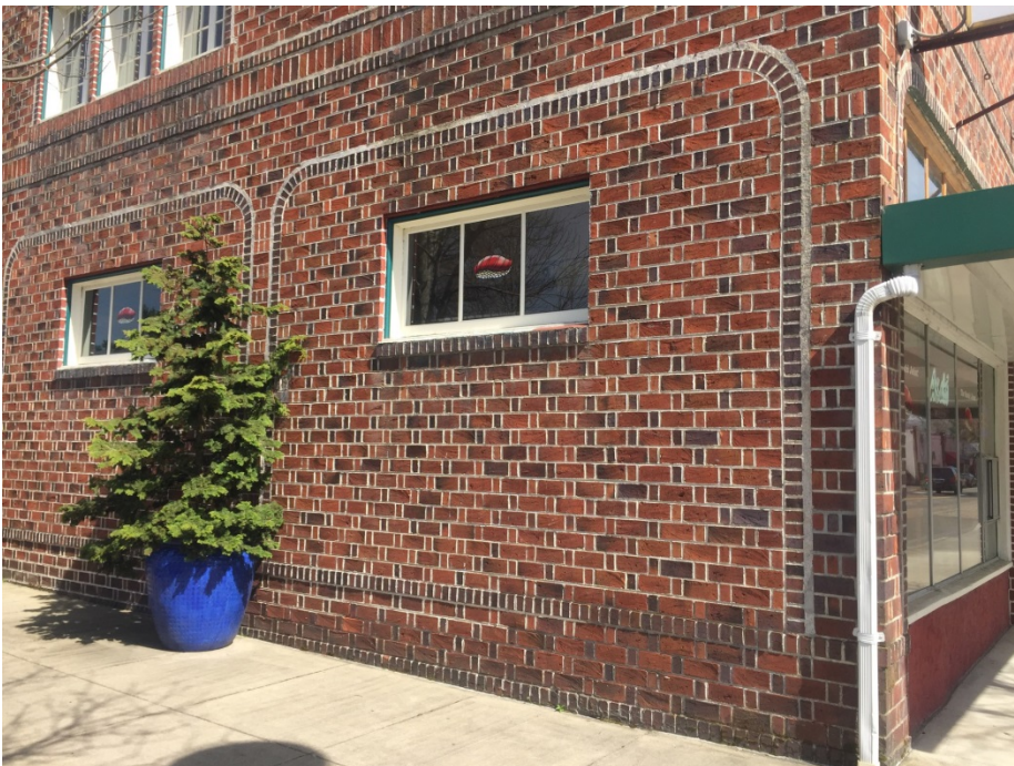
Photo 8: Detail of west façade showing first and second stories and brickwork
