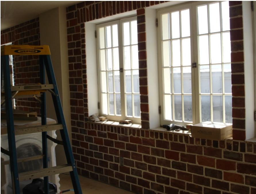
Photo 31: Second story – detail of typical window
