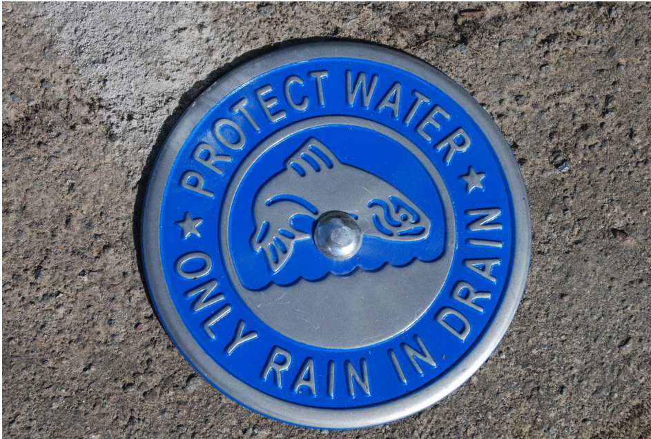
Storm drain medallion used to mark storm drains and catch basins
