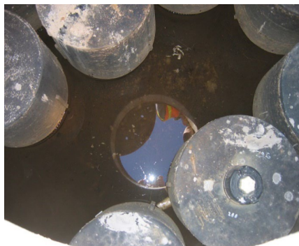
Filter vault cartridges
