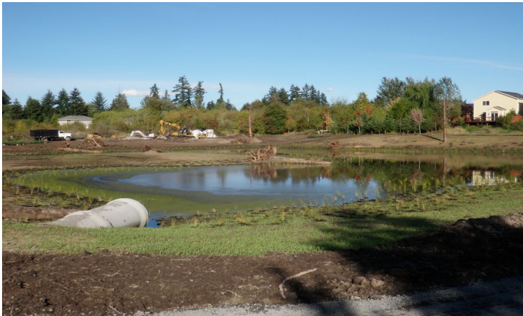
Construction of the Thomas Wetland East Stormwater Facility
