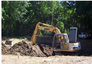
Excavator preparing land for a development.
