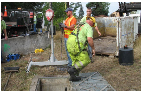
County crew replacing filters in a stormwater treatment filter vault system
