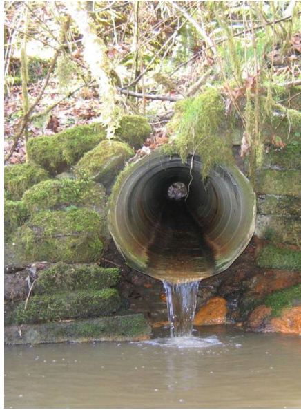
Culvert under a field road
