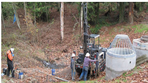
Encore stormwater facility retrofit
