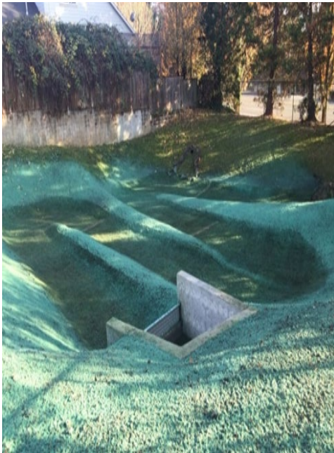
Recently reseeded stormwater facility biofiltration swale
