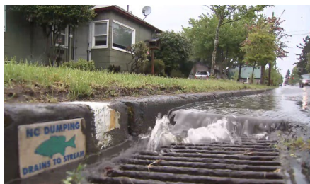
Typical residential catch basin
