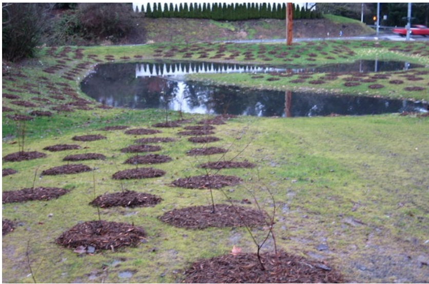
Stormwater facility with recently planted vegetation
