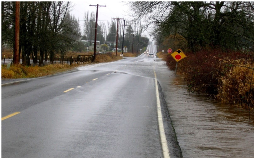
Roadway flooding during winter storm, 2007
