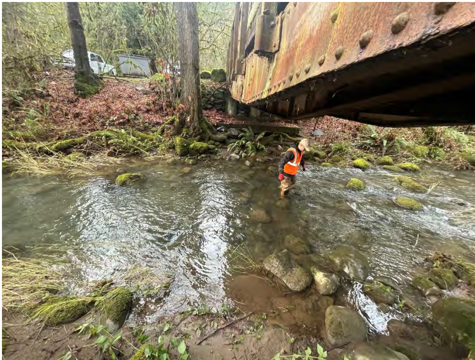
Stream under the bridge
