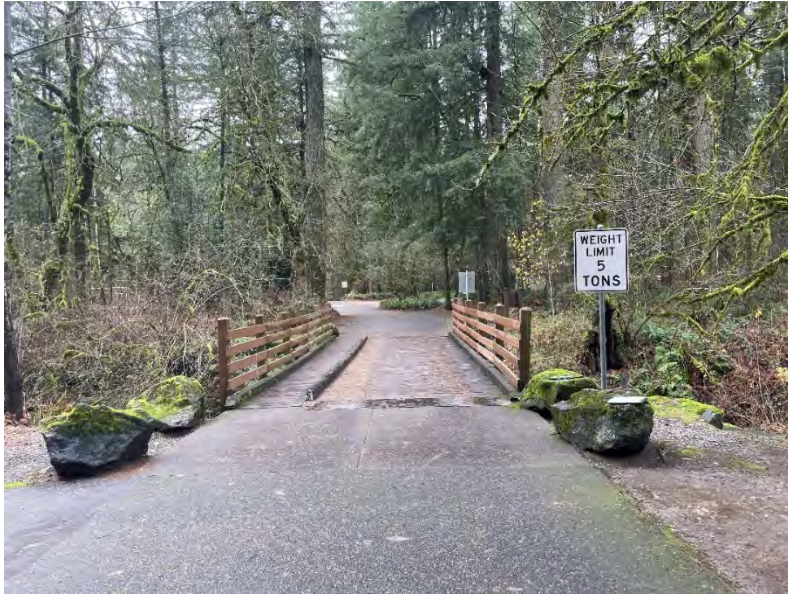
Photo 1, Lewisville No 1, Vehicle Bridge
