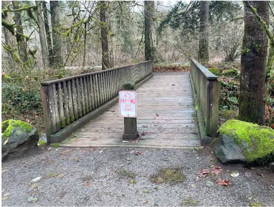
Photo 1 - Lewisville No 2 Approach and Deck view.
