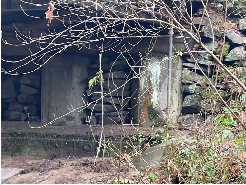
Photo 5 - Lewisville No 1 Rock filled spill through abutment with minor erosion.
