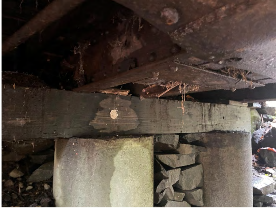
Photo 3 - Lewisville No 1 Timber Cap with rot and crush
