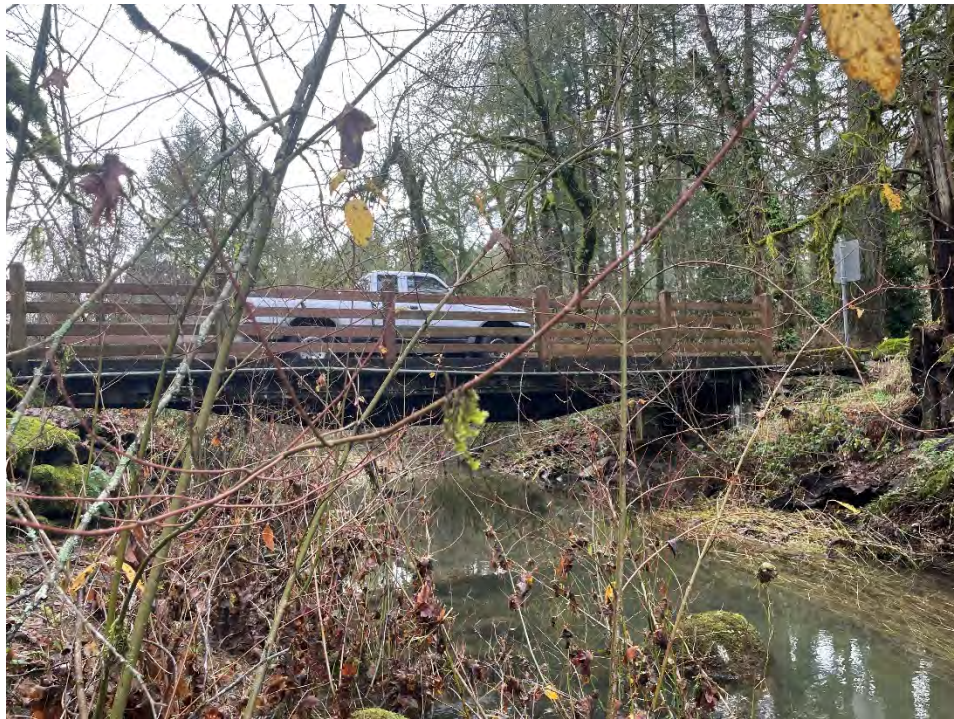
Photo 2 - Lewisville No 1 Elevation view.
