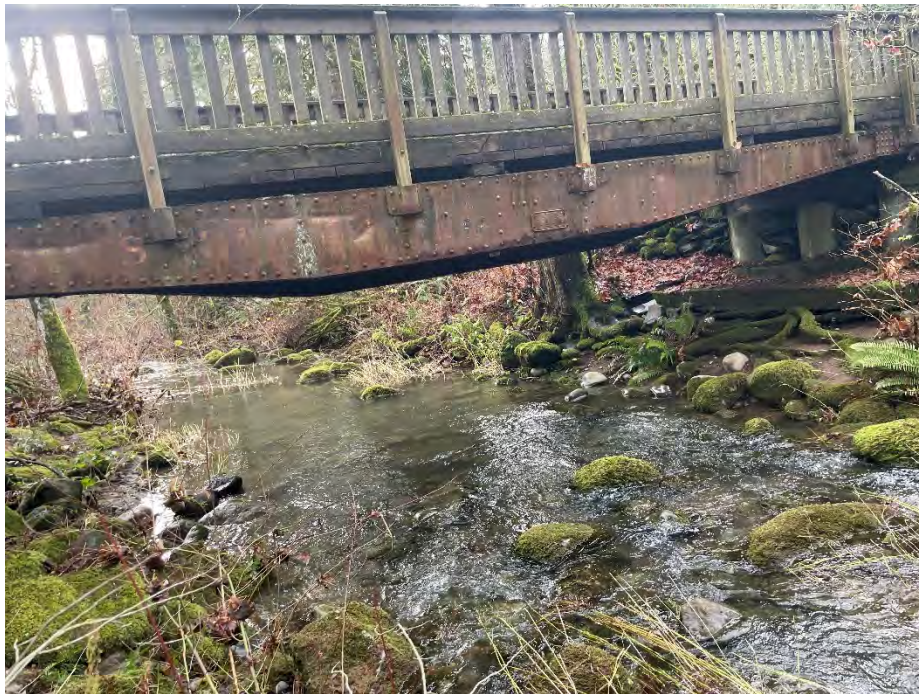
Photo 2 - Lewisville No 2 Elevation view.
