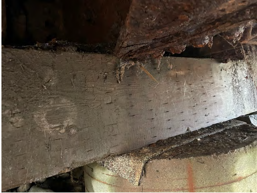
Photo 3 - Lewisville No 2 Timber Cap with rot and crush
