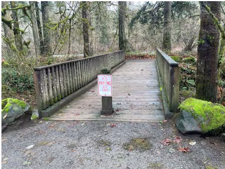
Photo 2, Lewisville No 2, Pedestrian Bridge
