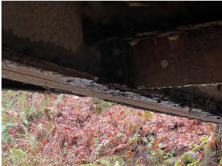
Photo 3 - Lewisville No 2 Timber Cap with rot and crush
