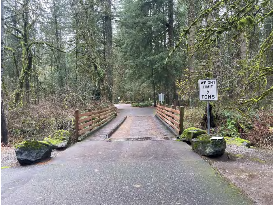
Photo 1 - Lewisville No 1 Approach and Deck view.
