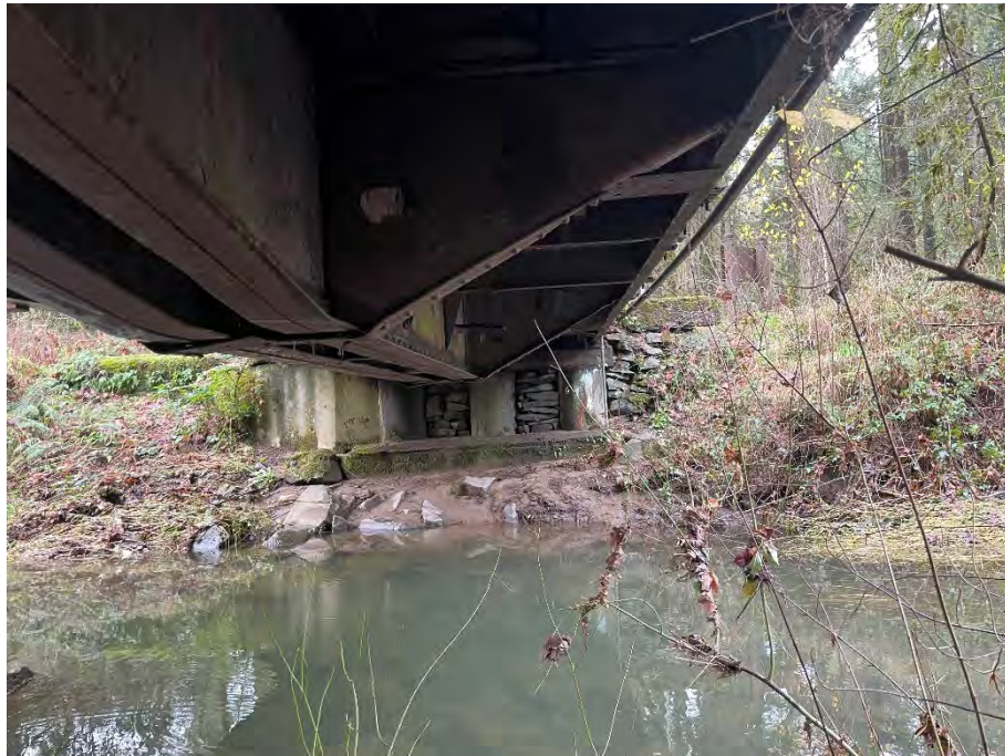
Photo 3 - Lewisville No 1 Timber Cap with rot and crush
