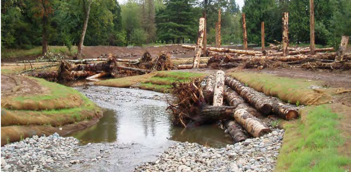
Figure 8: Example large wood and soil lift bank stability treatment that also improves channel complexity | Kelley Creek, WA.
