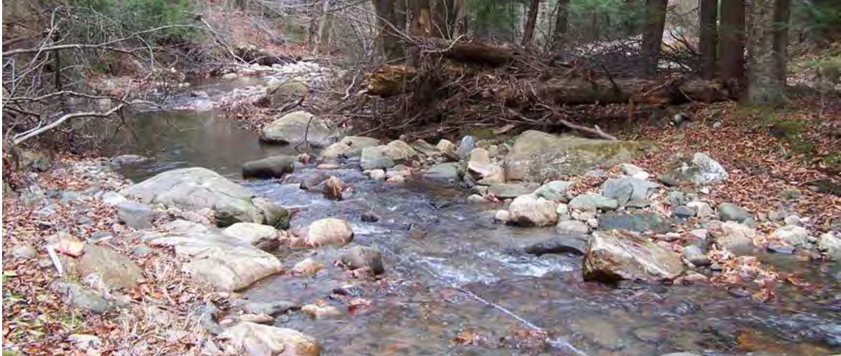
Figure 4: Series of rock steps installed for channel grade control | Tower Brook, Chesterfield, MA.
