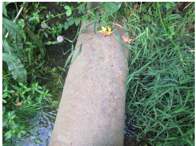
The photo on the left is taken looking downstream at a manhole at risk of bank erosion and exposure to channel hydraulics in Suds Creek. The photo on the right shows what we assume to be an exposed section of sewer line.
