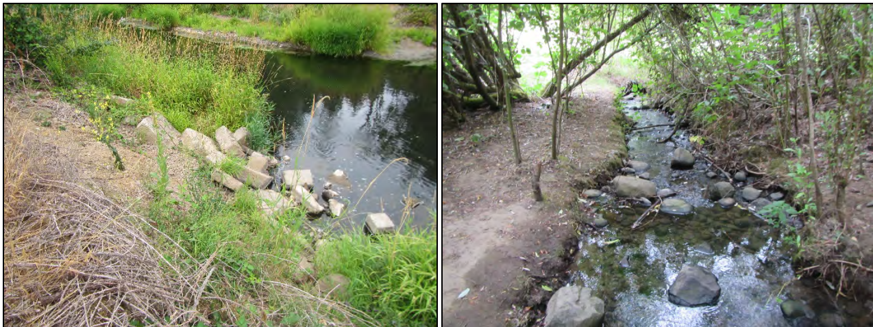
Floodplain disconnection, concrete bank riprap (left) and an incised, simplified channel lacking complexity and structures that slow and attenuate flow and sediment (right).
