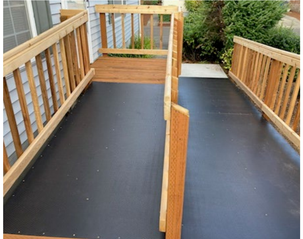
Front porch ramp after
