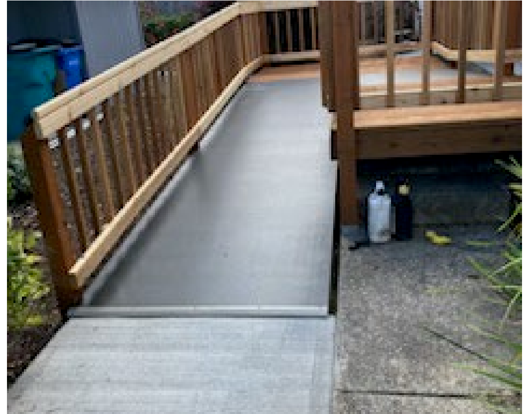
Sidewalk ramp after
