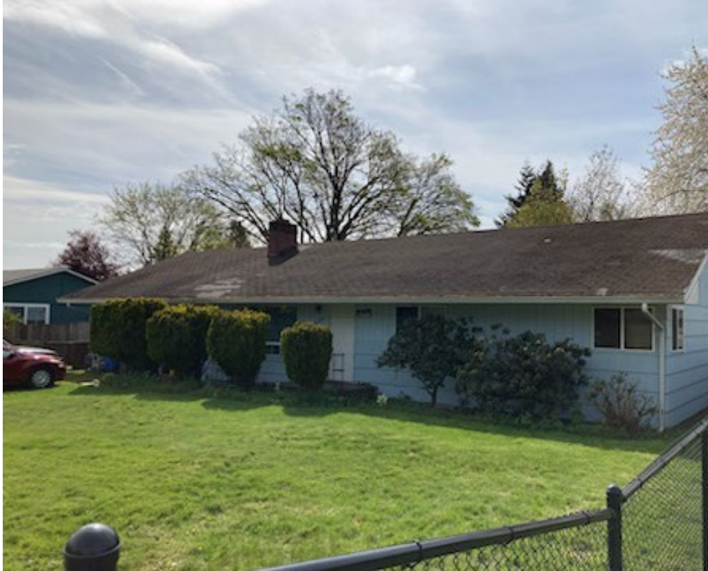
Roof repair before
