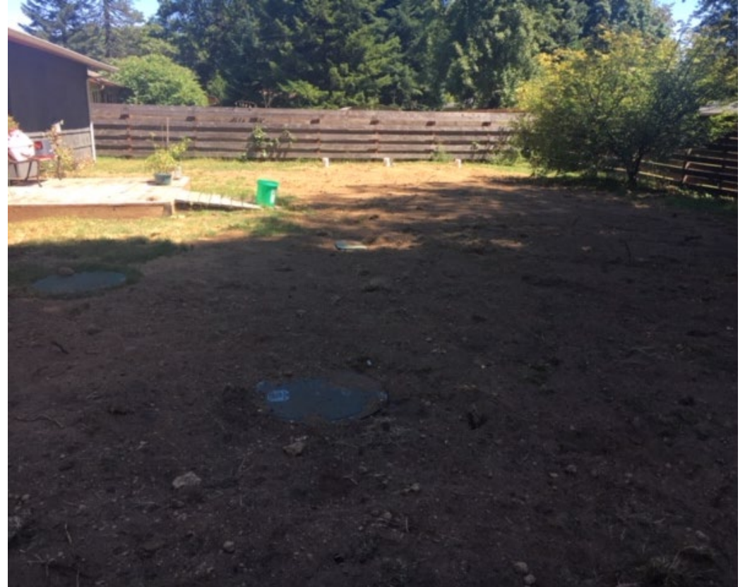
New septic and drain field after
