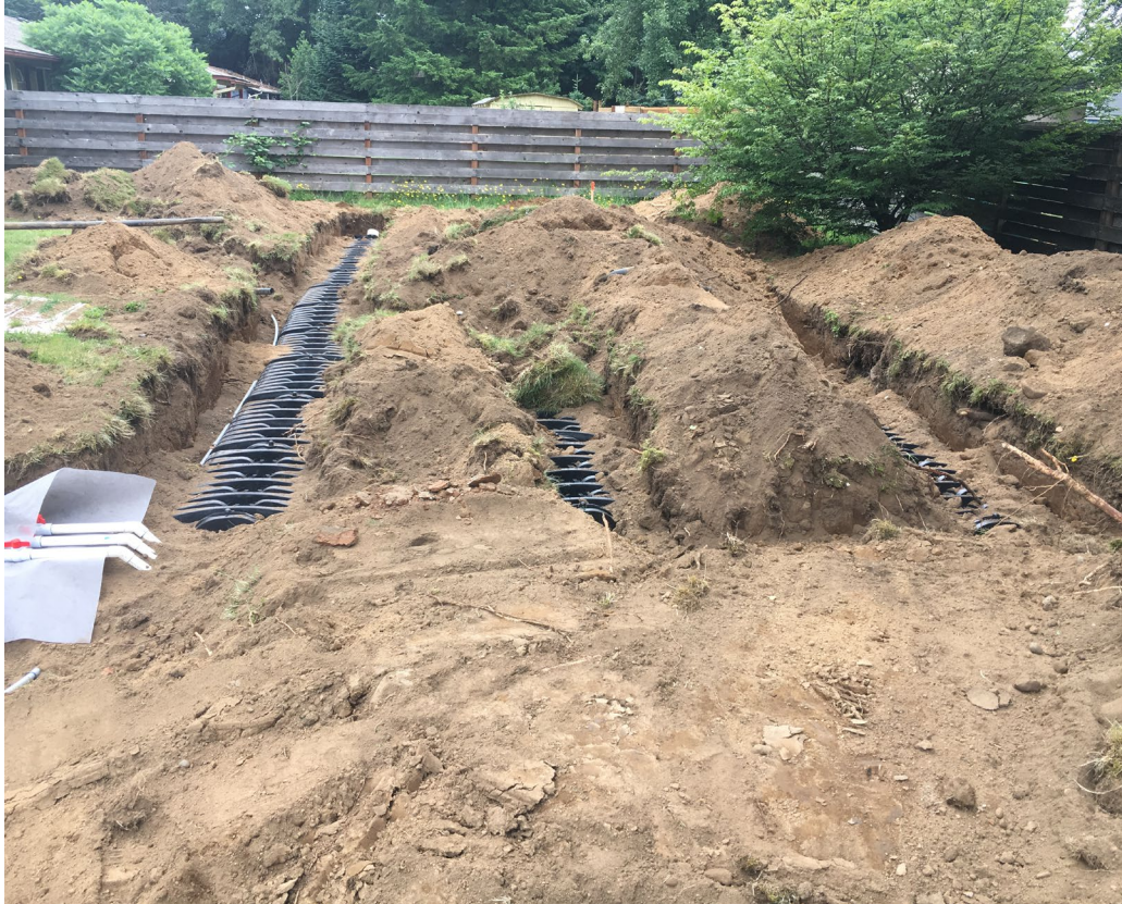
Septic drain field in progress
