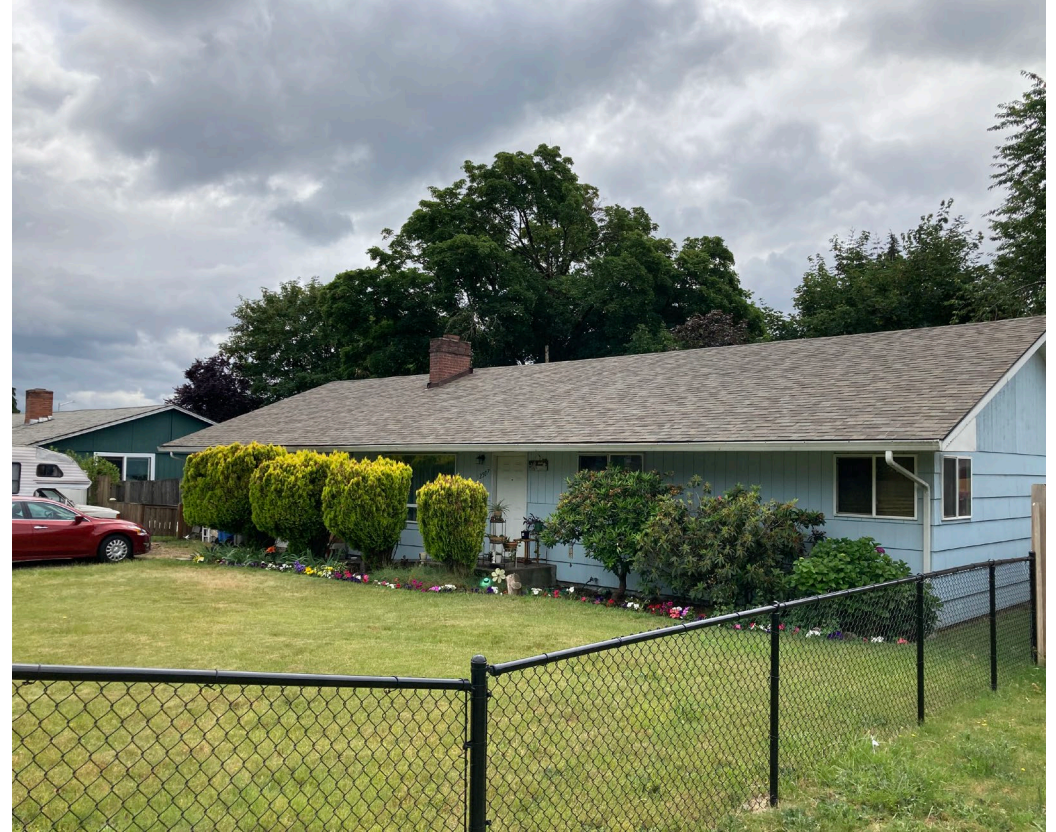
Roof repair after
