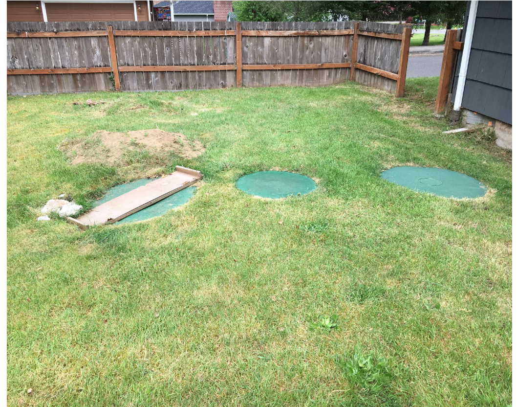
Backyard septic tanks before
