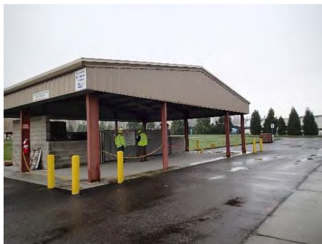
Figure 7: HHW Canopy and Concrete Slab
