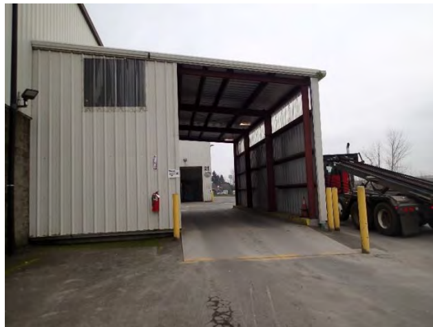
Figure 28: Used Oil Storage Facility
