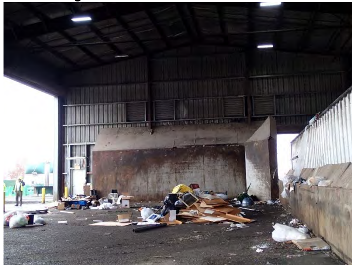
Figure 3: Structural Steel Frames
