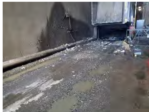
Figure 8 – Concrete Ramp in the Tunnel
