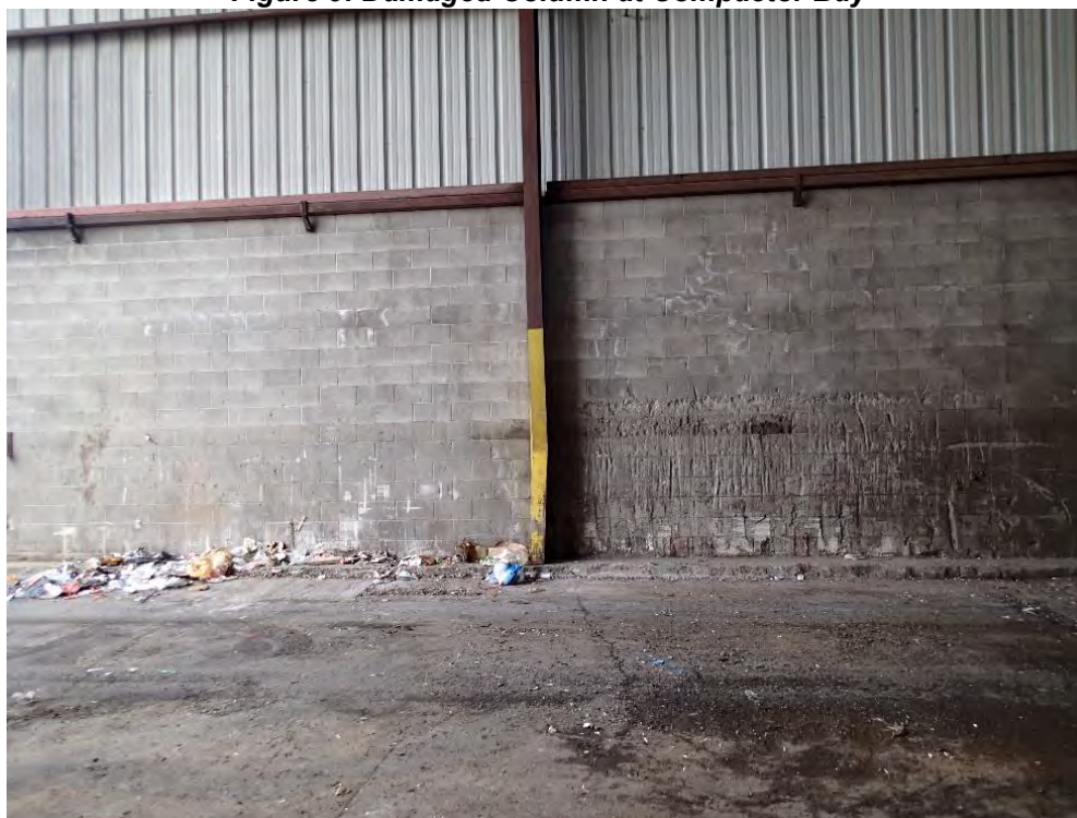
Figure 9: Damaged Column at Compactor Bay
