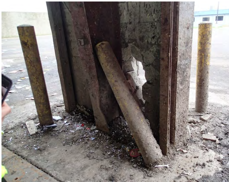
Figure 9: Damaged Column at Compactor Bay
