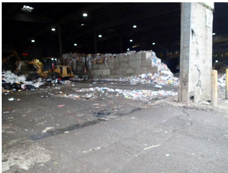
Figure 11: Concrete Floor in the Commercial Bays
