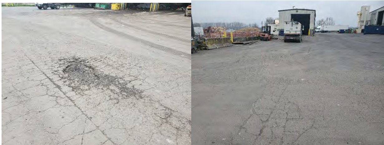
Figure 30: Upper Yard Pavement
