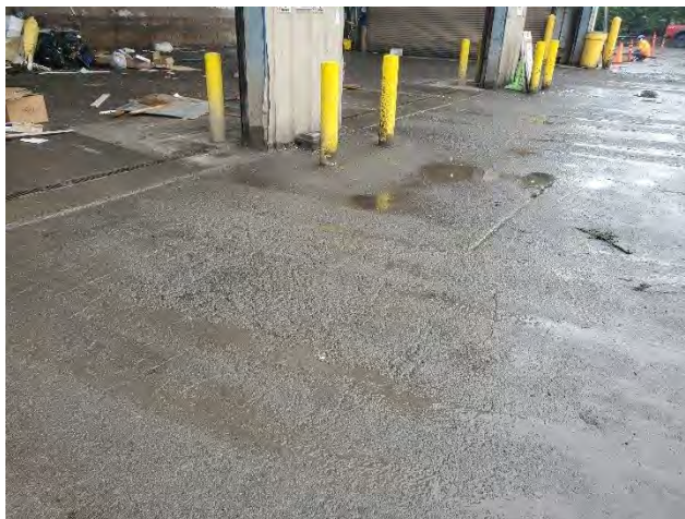
Figure 11: Paved Areas in Front of the Transfer Station
