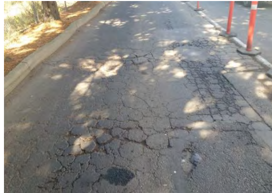
Figure 19 – Pavement Along Eastern Drive Aisle
