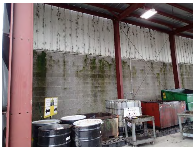
Figure 29: Interior of Used Oil Storage Facility
