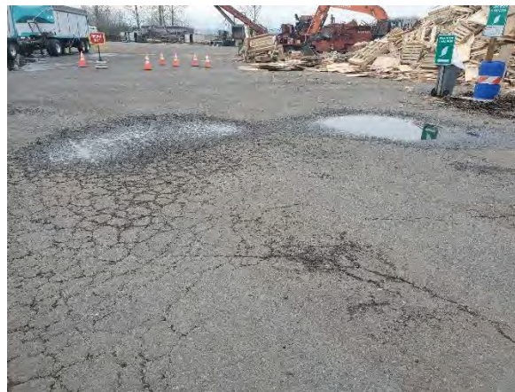
Figure 32: Lower Yard Pavement
