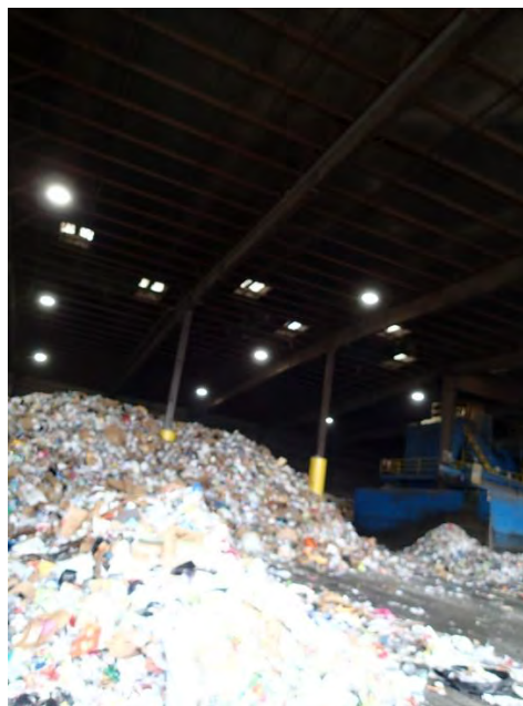
Figure 3: Recently Replaced Interior Columns with Concrete Encasement
