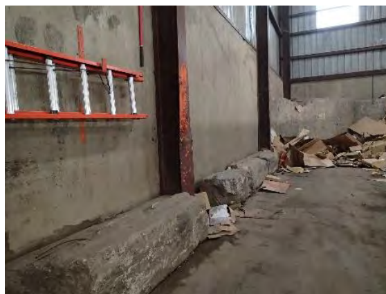
Figure 3 – Damaged Columns
