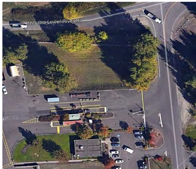
Figure 4.7: Entrance and Scale house Complex
