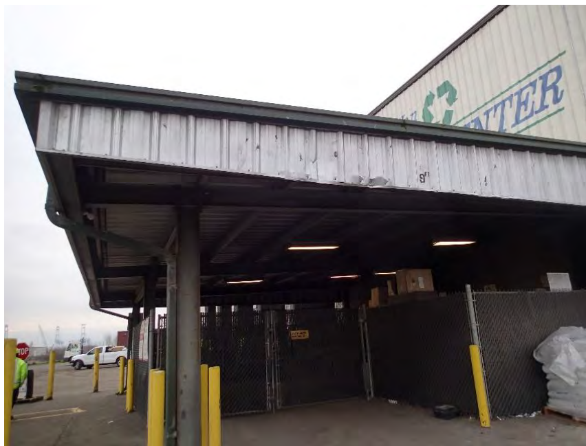
Figure 14: Damaged Siding
