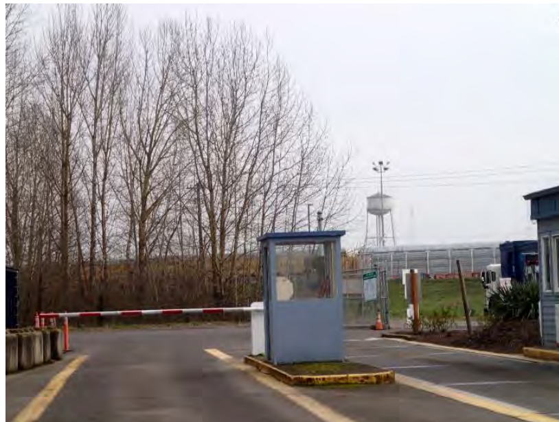
Figure 18: Scale House and Scales
