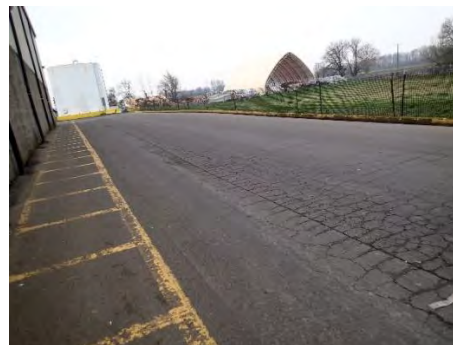
Figure 31: Paved Area North of Process Building
