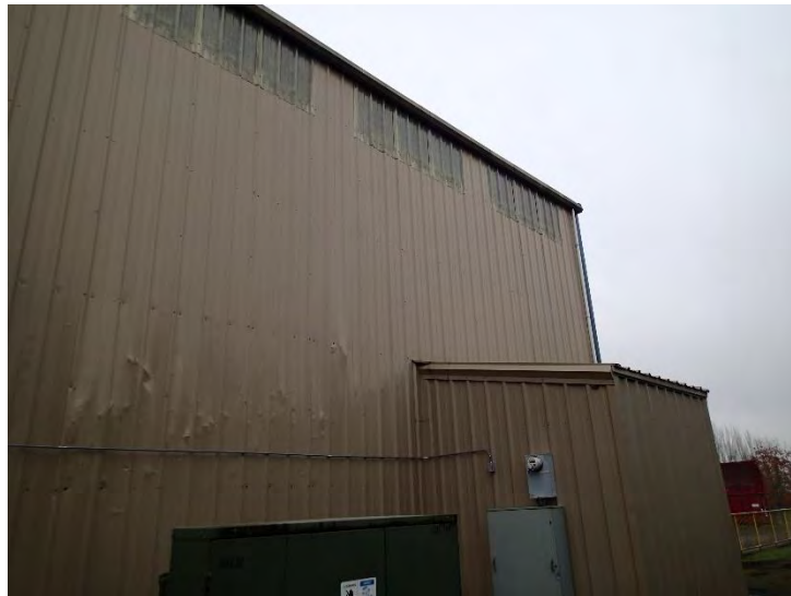
Figure 5: Damaged Siding
