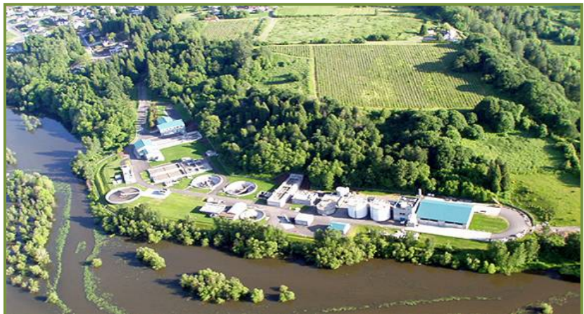
Salmon Creek Wastewater Facility
