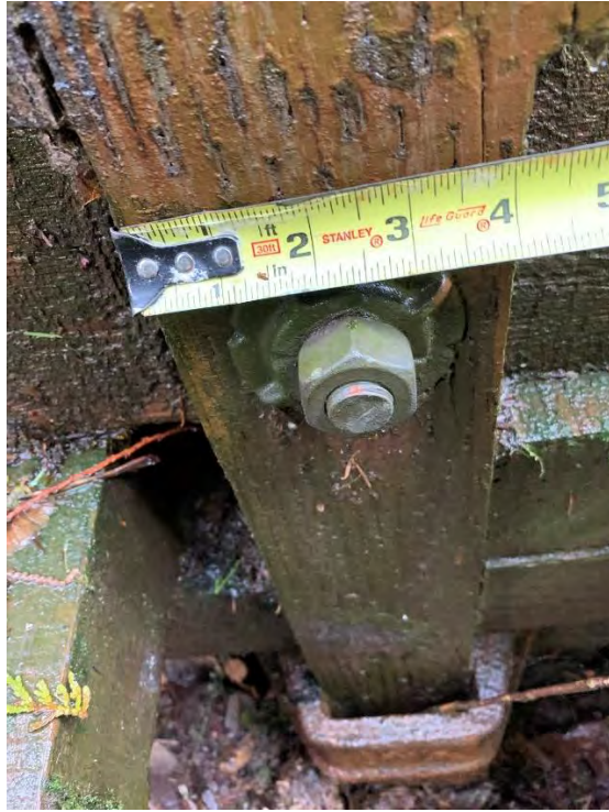
Photo shows railing and its bolted connection
