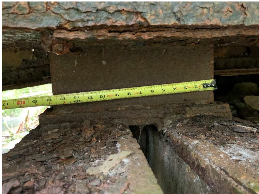
Photo shows the support diaphragm block
