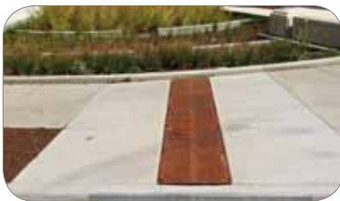
Stormwater management on site, not pipes
