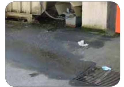
Pollution draining to stormwater system
